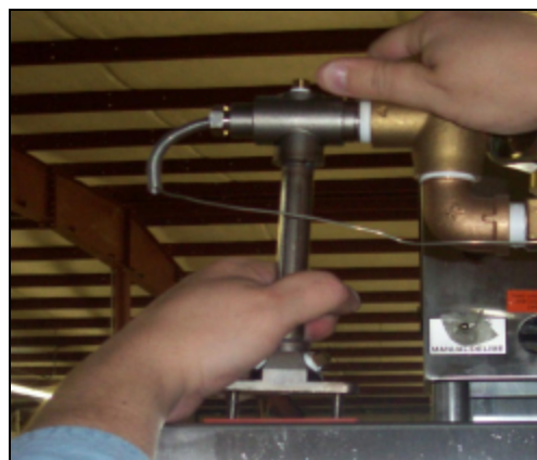
Lifting the rinse injector to make room
