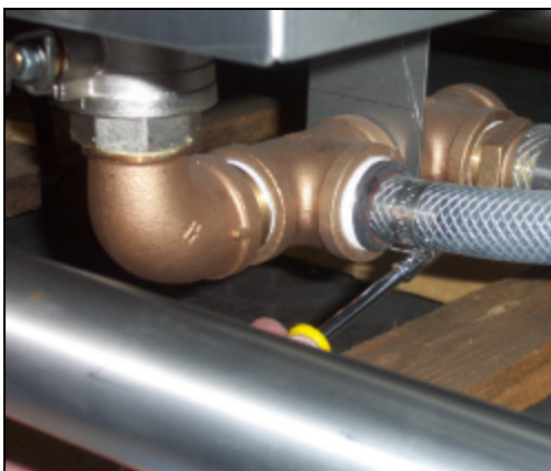
Loosening the rinse drain hose from the rinse drain nipple
