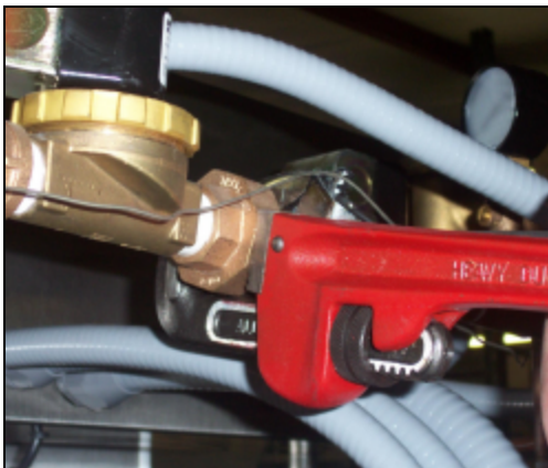
Loosening the union on the incoming plumbing
