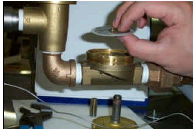
Removing the diaphragm
