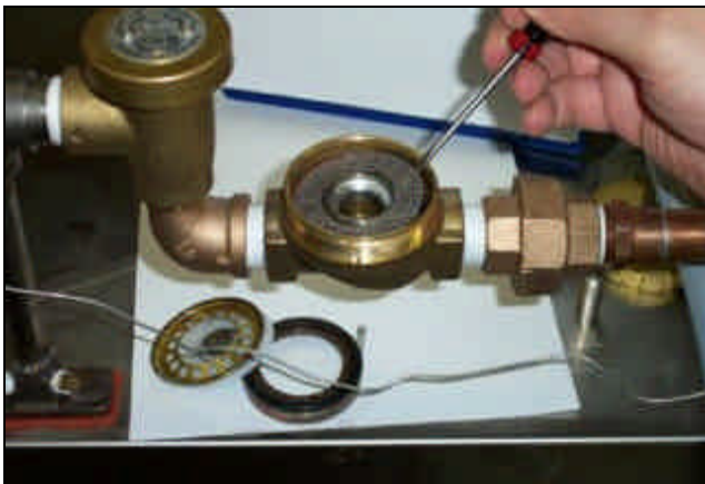
Removing the mesh strainer screen
