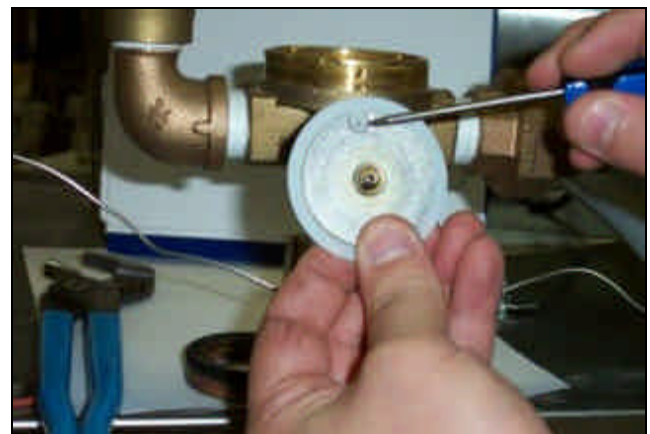
Pointing out the extension hole
