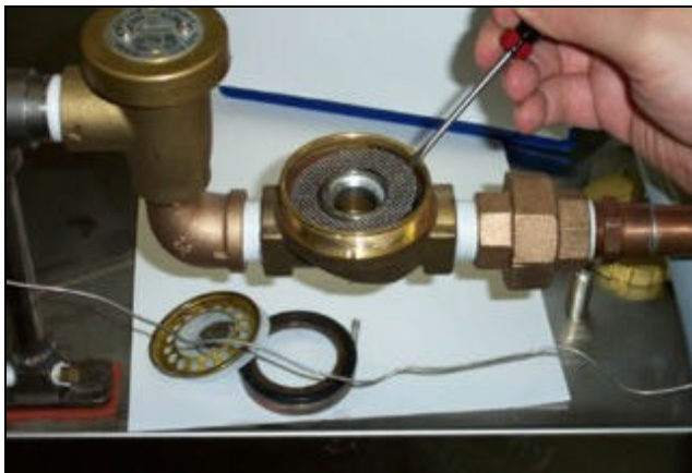
Removing the mesh strainer screen
