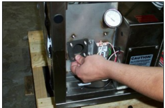
Removing the heater gasket
