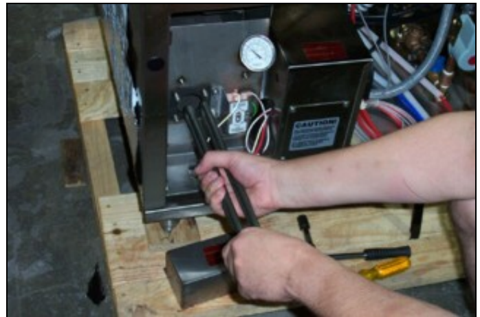
Pulling the heater out.
