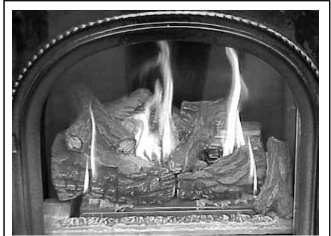
Figure 33 - Burner Flame Appearance
