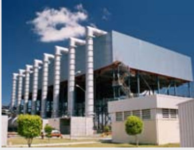
Rio Bravo Chihuahua, Mexico — ACC for 3 x 515 Combined Cycle Power Plant
