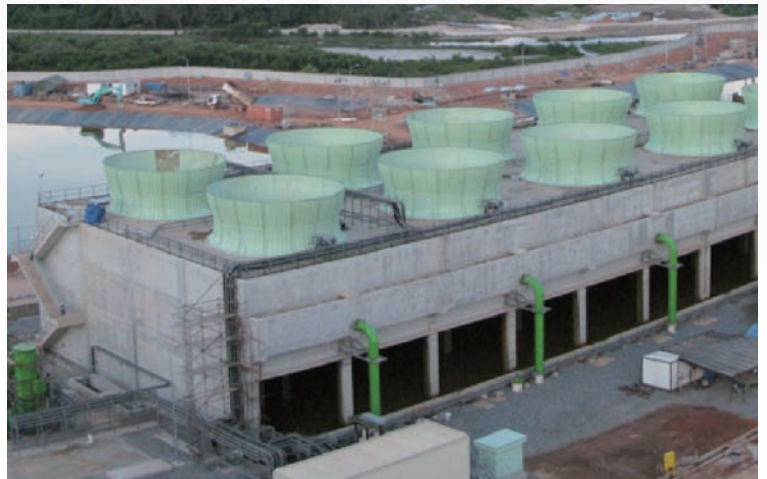
Class 800 cooling towers in Thailand
