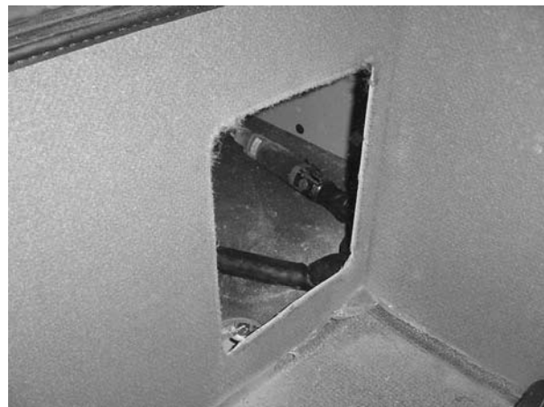
Figure 7 - Return air vent hole cut
