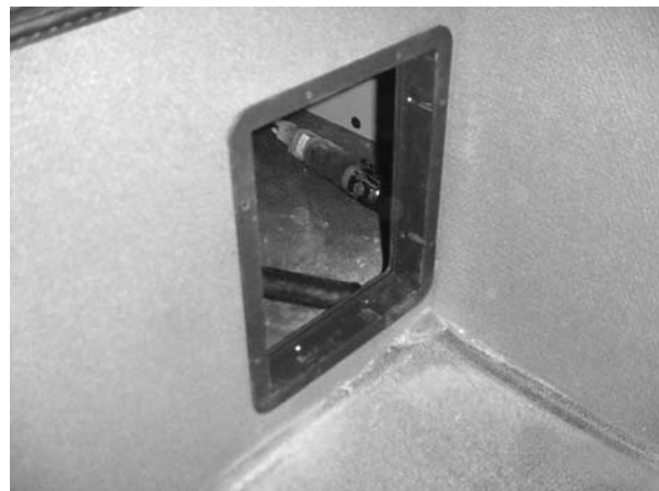
Figure 8 - Return air grill flange installed
