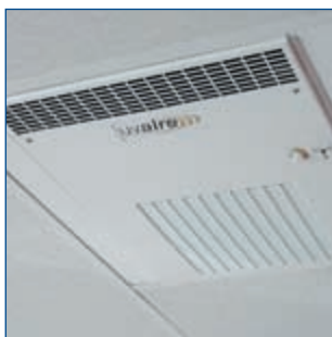
Drop ceiling installation
