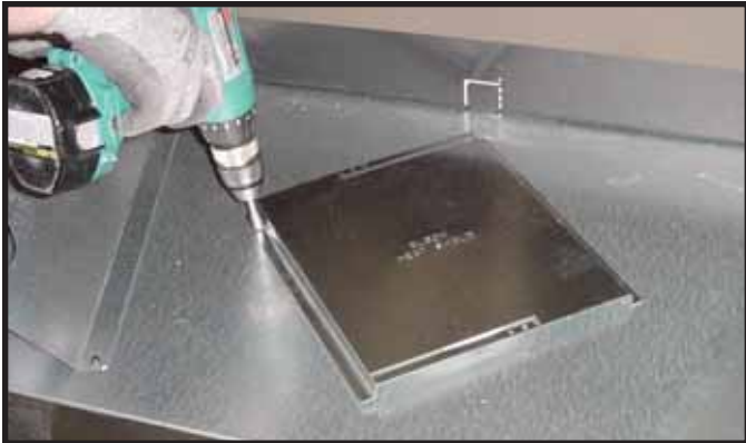
Figure 7.1 For top vent, remove the two screws holding the elbow heat shield in place. Use this heat shield over the first elbow if applicable. For rear vent skip this step.
