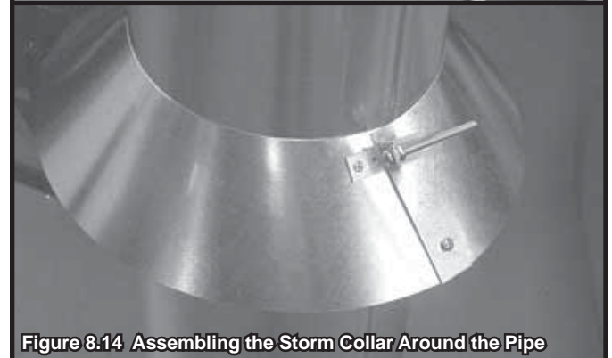
Figure 8.13 Assembling the Storm Collar
