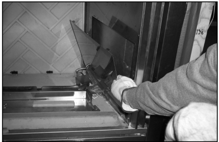
Figure 6.4 Remove Valve Access Panel
