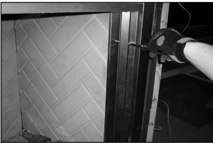
Figure 12.3 Loosen Refractory Retaining Strip
