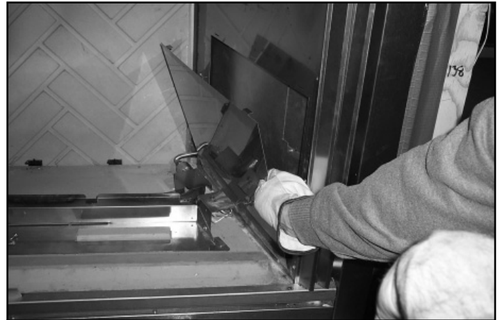
Figure 12.4 Remove Valve Access Panel
