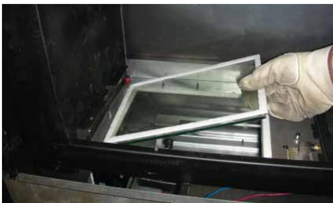
Figure 12.13. Removing Glass Pane Frame.
