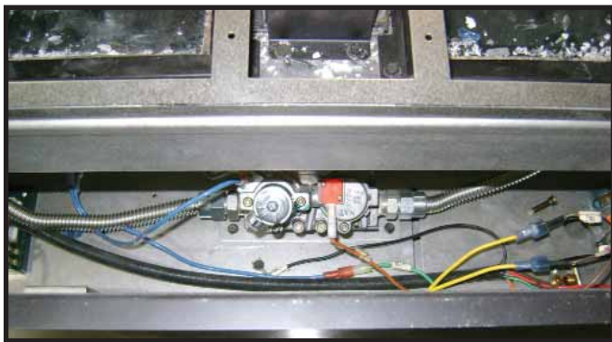
Figure 11.1. Valve Pressure Taps.
