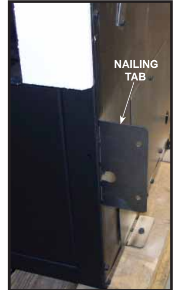
Figure 9.4 Nailing Tabs Installation Position
